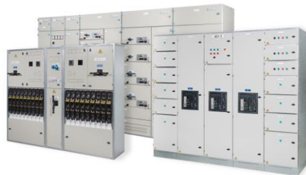
HEMP, 8HS, 8PU, 8PT LV Power Distribution Boards
